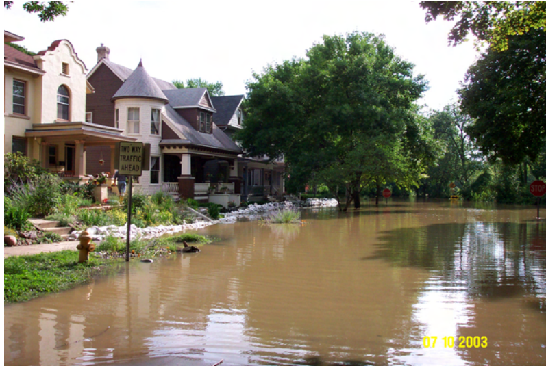
Homes in the West-central neighborhood are protected with sandbags lined up along the sidewalk. Flood-damages in this area are mostly limited to water in basements. The builders had the foresight to construct these homes high enough to endure a flood matching the 1913 levels.
