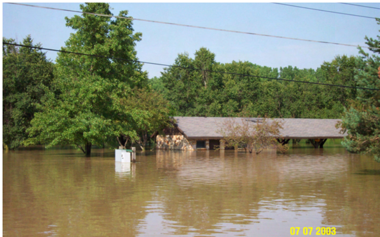
Kekiong Park pavilion yields to St. Marys River Floodwater.
