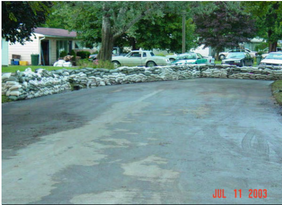
Thousands of sandbags block the floodwater from reaching homes in the Belle Vista neighborhood. The local residents “know the drill” as they have been through this experience many times.
